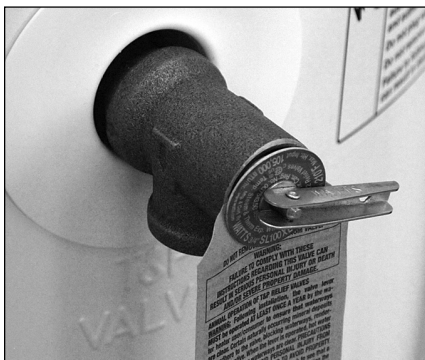
Figure 25 - Temperature and Pressure Relief Valve
