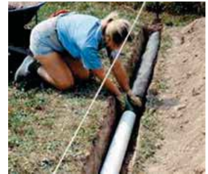
Figure 65: Underground Refrigerant Piping.
