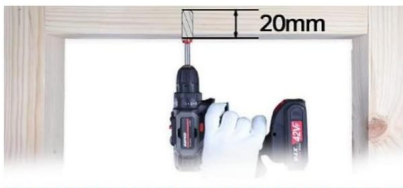
Use Wood Drill Bit Dia 1/2" at the top
