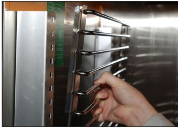
Fig. 7b. Installing kit #2 rod tray sides.
