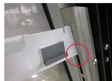
Bottom notch installed (no gap)
