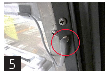
Light cord installed
