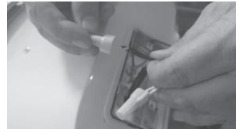
Figure 18 - Connecting the electrical wires.
