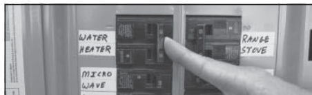
Figure 27 - Circuit Breaker
