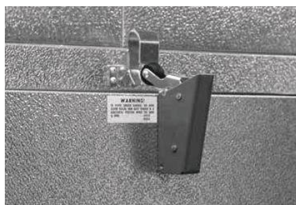
Roller Too High
