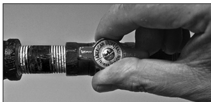
Figure 32 - Gas valve in "on" position
