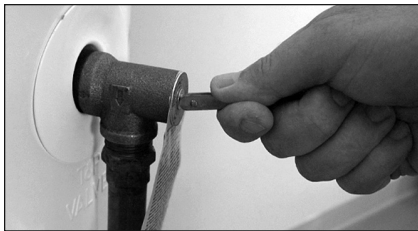
Figure 43 - T&P Relief Valve.
