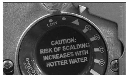
Figure 37 - Adjust the gas control knob to "▲".
