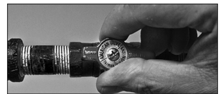
Figure 50 - Gas valve in "on" position.
