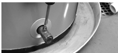
Figure 40 - Draining the water heater.
