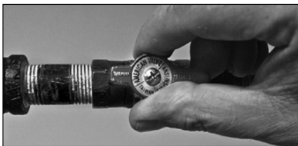
Figure 33 - Gas valve in "on" position
