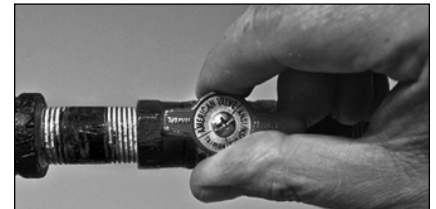
Figure 51 - Gas valve in "on" position.
