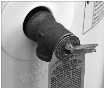
Figure 25 - Temperature and Pressure Relief Valve
