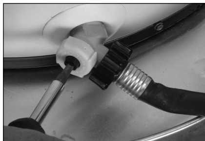
Figure 20 - Draining the old water heater.
