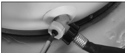
Figure 41 - Draining the water heater.
