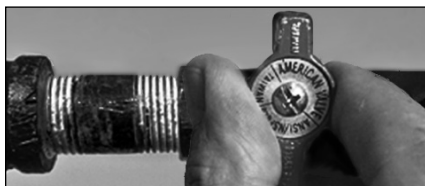
Figure 47 - Gas valve in "off" position.
