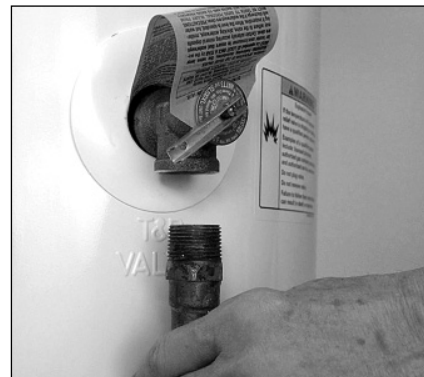
Figure 21 - Removing the T&P Relief Valve discharge pipe.
