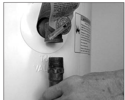
Figure 20. Removing the T&P Relief Valve discharge pipe.
