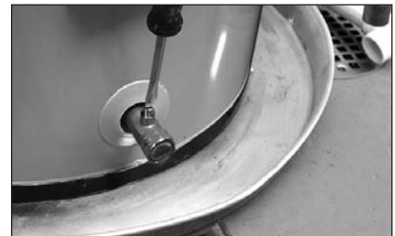
Figure 19. Draining the old water heater.
