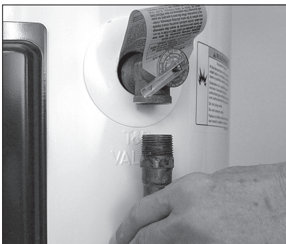
Removing the T&P Relief Valve discharge pipe.
