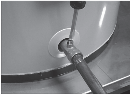
Draining the old water heater.
