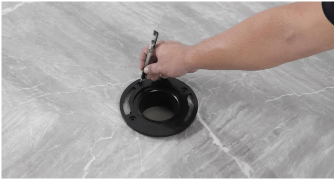
2. Place the fixed disk into the drain outlet and mark the screw hole positions.
