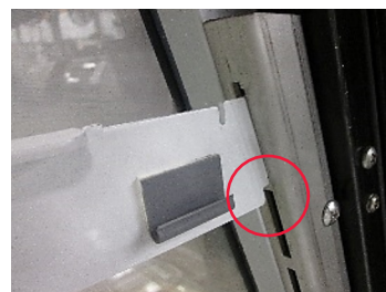
Top notch installed (gap)
