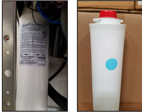
Filter Label Location
