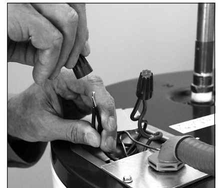
Figure 19 - Connecting the electrical wires.
