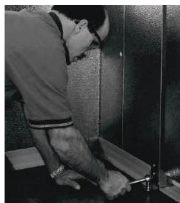
Attach slam brace with fastener provided
