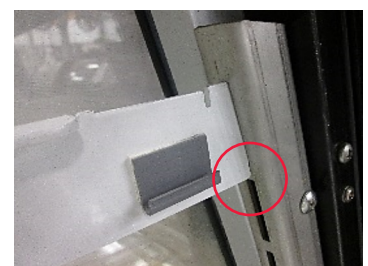
Bottom notch installed (no gap)
