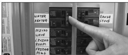
Figure 42 - Circuit Breaker.
