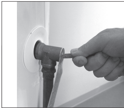
Figure 49 - T&P Relief Valve.
