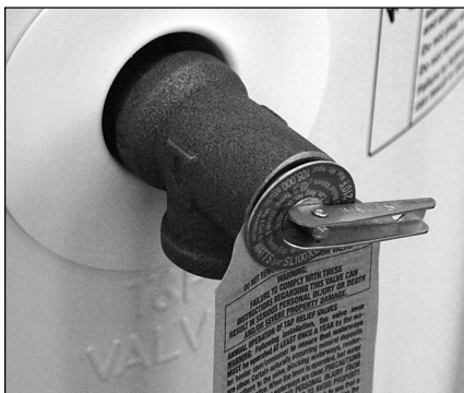
Figure 25 - Temperature and Pressure Relief Valve
