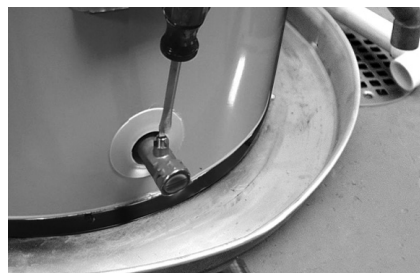
Figure 20 - Draining the old water heater.
