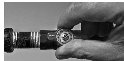
Figure 58 - Gas valve in “on” position.
