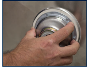
3. Screw on Die Cast Nut and Tighten
