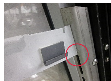
Bottom notch installed (no gap)
