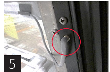
Light cord installed
