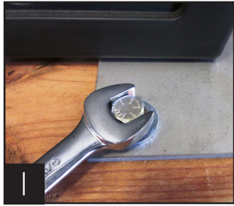
1 Removing bracket from skid.
