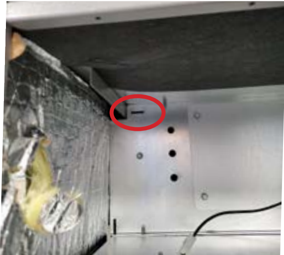
Figure 5. Notch for Control Panel Relocation
