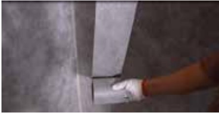
Cover the waterproofing strip on the corner
