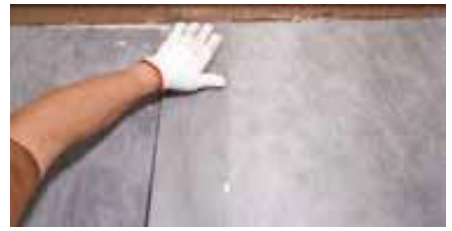
Cover the waterproofing strip on the joint
