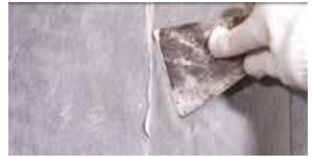
Make the wall surface even
