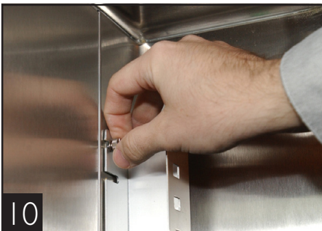
Pilaster installation (side wall of cabinet)
