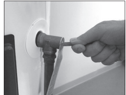
Figure 38 - T&P Relief Valve
