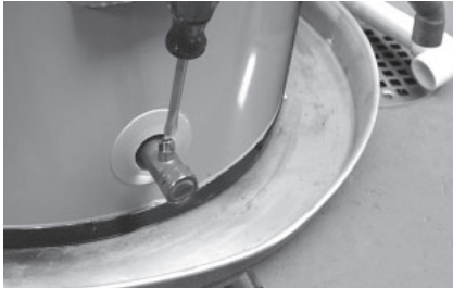
Figure 10 - Draining the old water heater.
