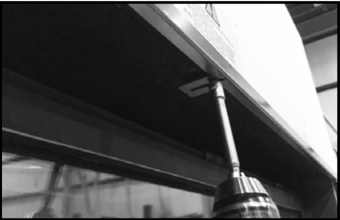
Figure 10.5 Install Trim Ring
