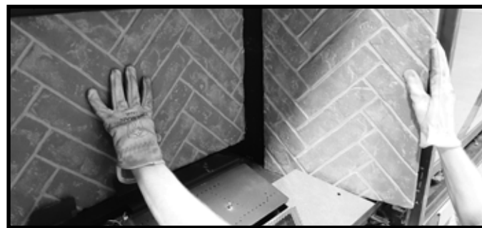
Figure 11.3 Install Side Refractory Panel (Right Side Shown)
