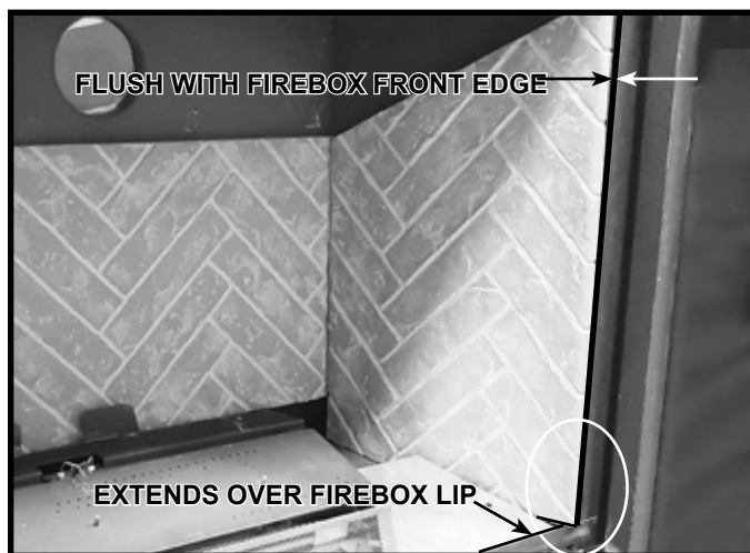
Figure 11.4 Side Refractory Panel Installed (Right Side Shown)
