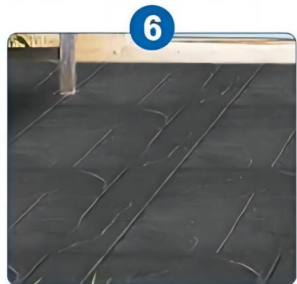
Spray sealing protective agent
