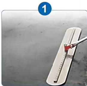
Screeding the concrete
