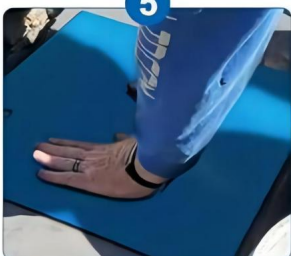
Stamp the concrete
