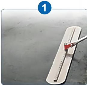
Screeding the concrete
