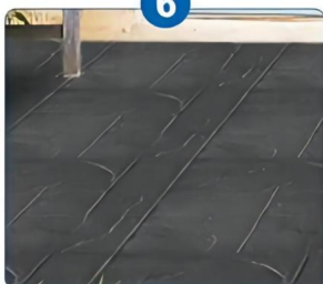
Spray sealing protective agent
