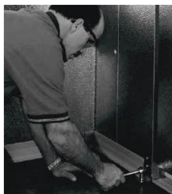
Attach slam brace with fastener provided
