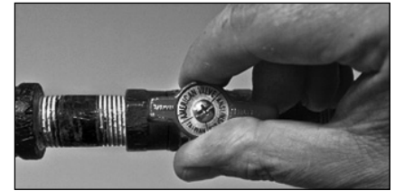
Figure 42 - Gas valve in "on" position.
