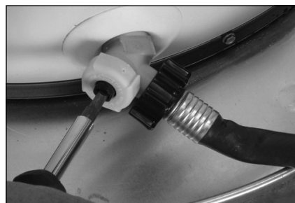
Figure 19 - Draining the old water heater.
