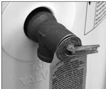
Figure 22 - Temperature and Pressure Relief Valve
