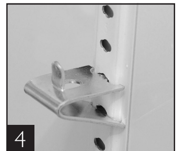
4 Shelf clip installation complete
