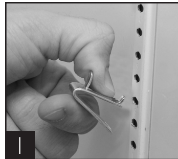
1 Installing top tab of shelf clip
