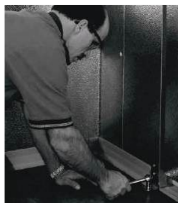
Attach slam brace with fastener provided
