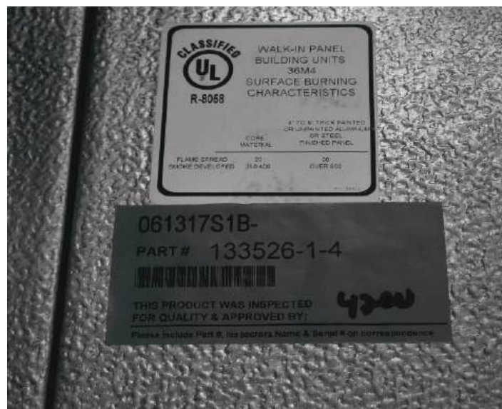
RSG Inspection Label and Panel Specific Part Number
