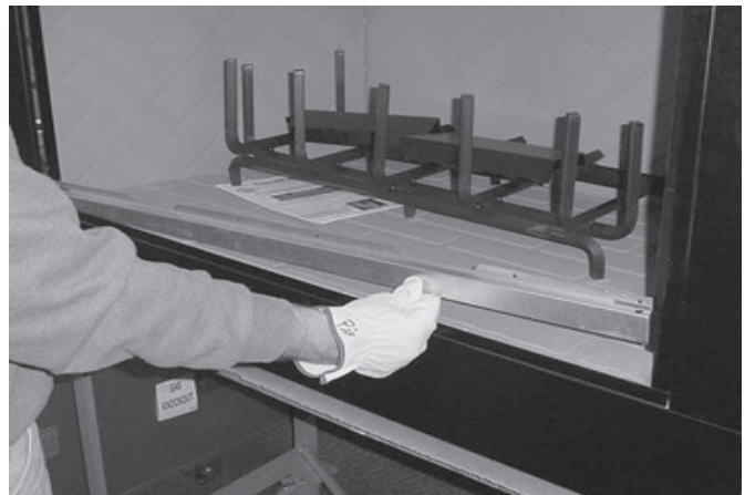
Figure 1 - Install the Door Track
