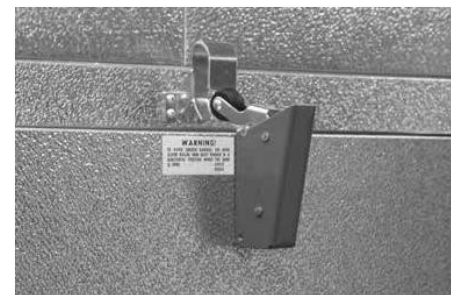
Roller Too High
