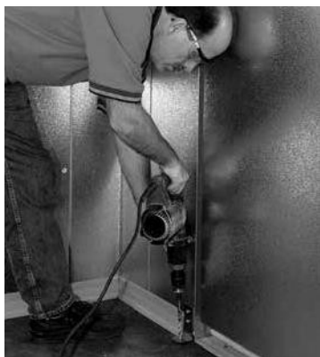
The recommended hole size for PARABOLT ANCHOR is 3/8" X 2-1/4"
