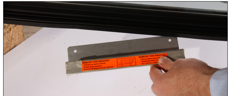
Fig. 2. Remove the glass swing door shipping bracket, if so equipped. Do not discard.
