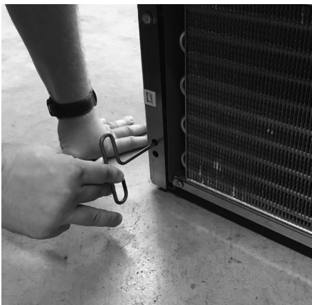
Adjusting rear leveling legs.
