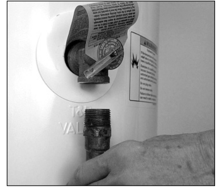
Figure 21 - Removing the T&P Relief Valve discharge pipe.
