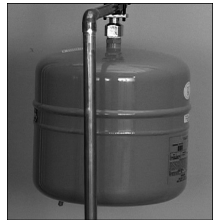
Figure 13 - A Thermal Expansion Tank helps protect the home's plumbing system from pressure spikes.
