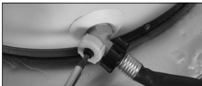
Figure 42 - Draining the water heater.
