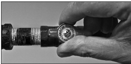
Figure 32 - Gas valve in "on" position
