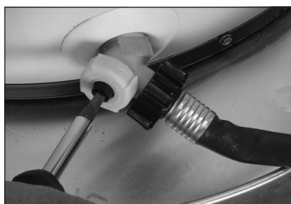
Figure 20 - Draining the old water heater.
