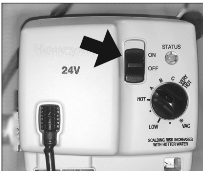
Figure 37 - Turn gas control/temperature knob OFF.
