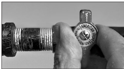
Figure 45 - Gas valve in "off" position.
