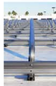
One Common Bolt for All Joints
