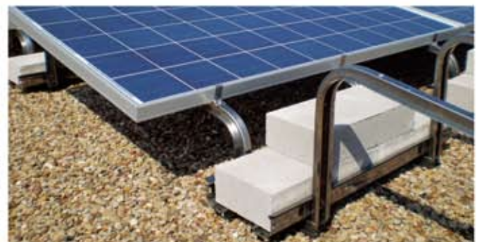
Panel Clamps with Integrated Grounding
