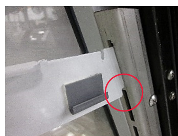
Top notch installed (gap)
