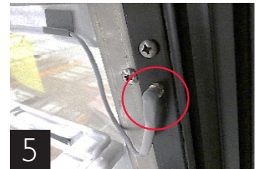
Light cord installed
