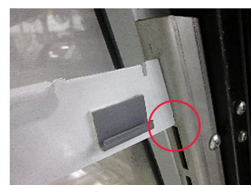
Bottom notch installed (no gap)
