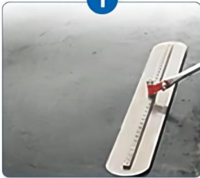
Screeding the concrete
