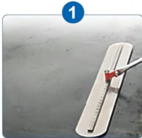
Screeding the concrete
