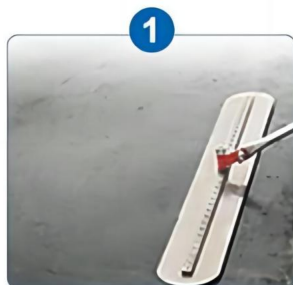
Screeding the concrete
