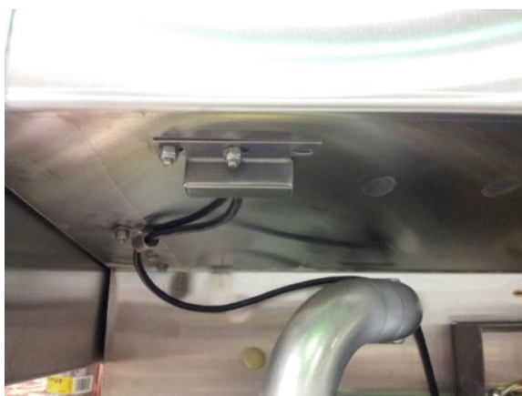
Sequence reed switch for wash tank
