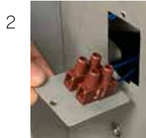
WITH OUT BRIDGE 240V
