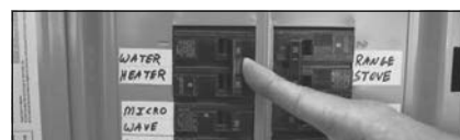
Figure 38 - Circuit Breaker
