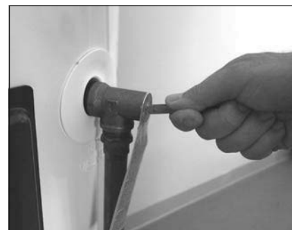
Figure 46 - T&P Relief Valve
