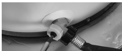
Figure 26 - Drain Valve
