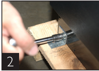
Removing bracket from cabinet.
