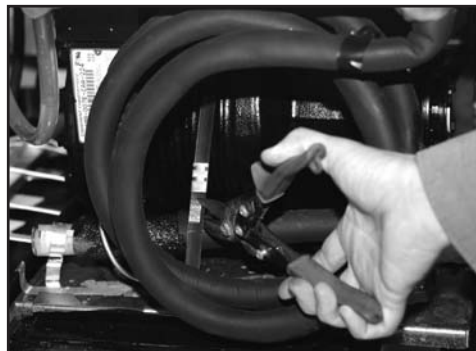
Cutting band that is around compressor
