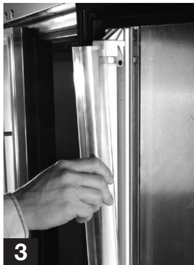
3 IDL (Integrated Door Lighting)
