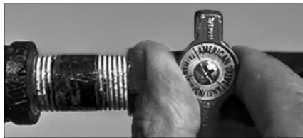
Figure 47 - Gas valve in “off” position.
