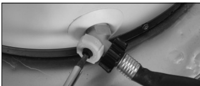
Figure 41 - Draining the water heater.
